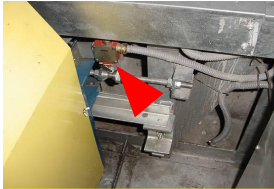
Broken Step Chain Safety Device
