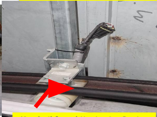
Handrail Speed Monitoring Device
